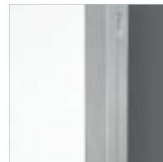
Door leaf rebate protected with stainless steel profile
